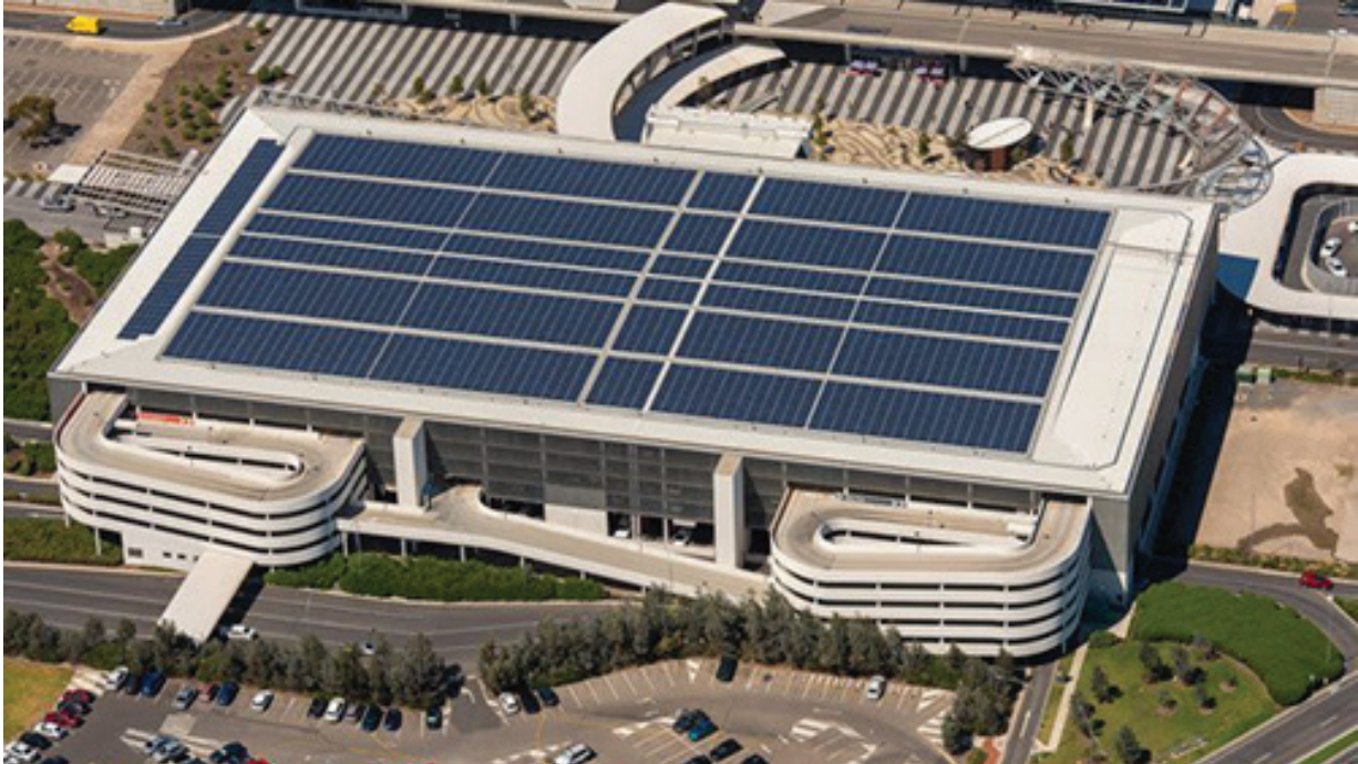
The rooftop of the Adelaide Airport car park covered in solar panels -
